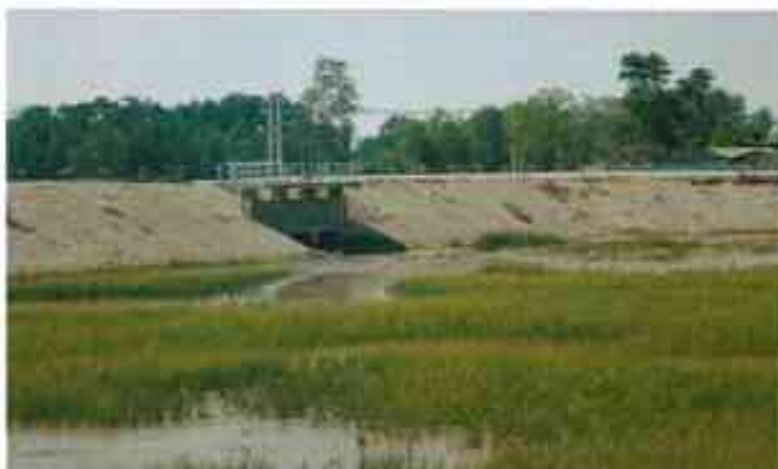
Figure 7. Condition of SW-1 and its surrounding
