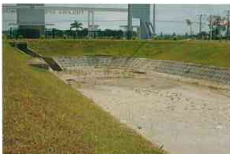
Figure 8. Condition of SW-5 and its surrounding
