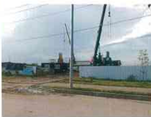
Figure 2 Construction Site near around the box culvert.
